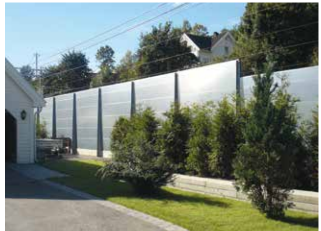
Noise and privacy panels along railway, Oslo, Norway.
