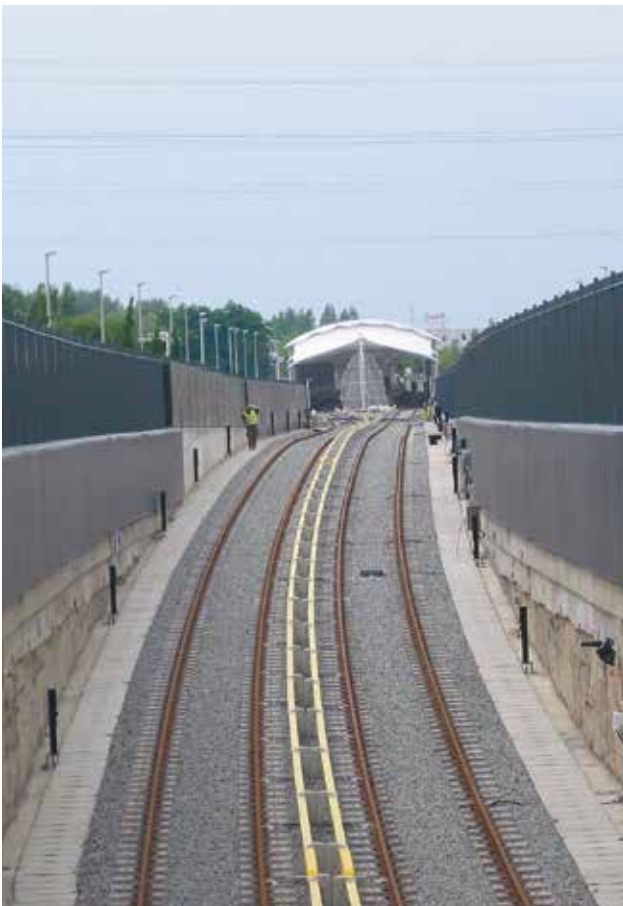
Noise panels at underground descent, Brussels, Belgium.
