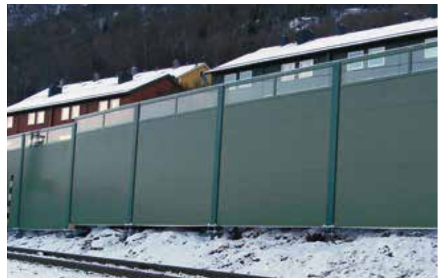
Noise-absorbing panels with glazing, Narvik, Norway. (NOTE: 4 m between posts).
