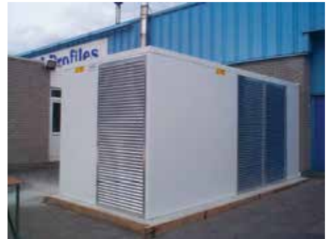
Noise enclosure, D J Profiles Ltd, Telford, England.
