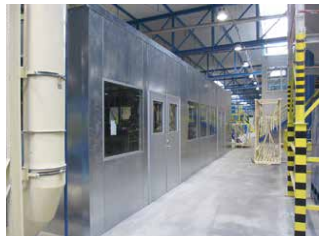
Noise enclosure, Teplice, Czech Republic.
