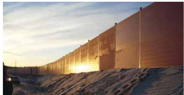
Noise panels along highway E10 at discharge station for iron ore, Svappavaara, Sweden.
