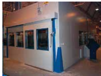
Noise enclosure, automated punching machinery, Bristol, England.
